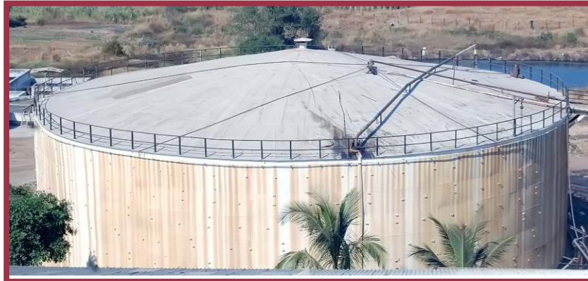
MOLASSES STORAGE TANKS
